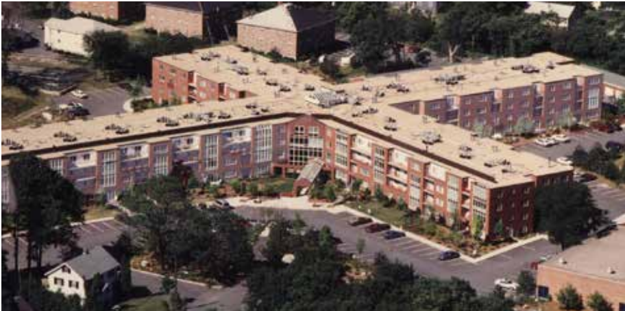
The 147-unit Place Lane Condominium in Woburn, Massachusetts, with the original Woburn Boys Club swimming pool and gym shown next door in the lower right corner
