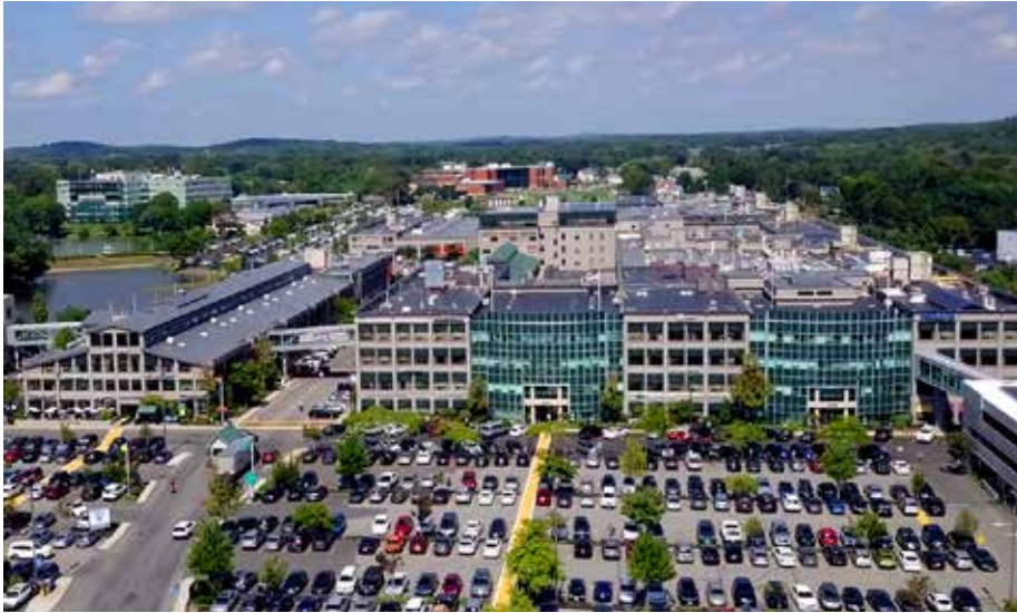
| A view from the south of a booming 2-million-square-foot Cummings Center
