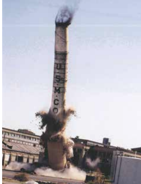
| Implosion of The Shoe's 225-foot-tall chimney
