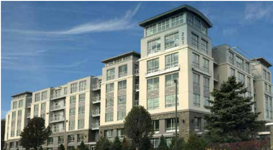
| Elliott Landing condominiums at Cummings Center, Beverly, 2019
